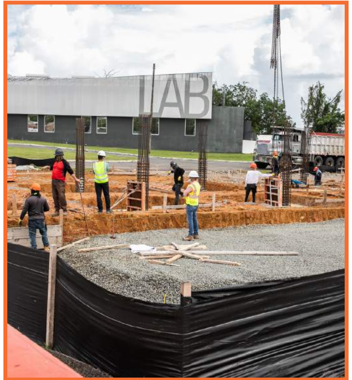
Forward Center Construction Process
