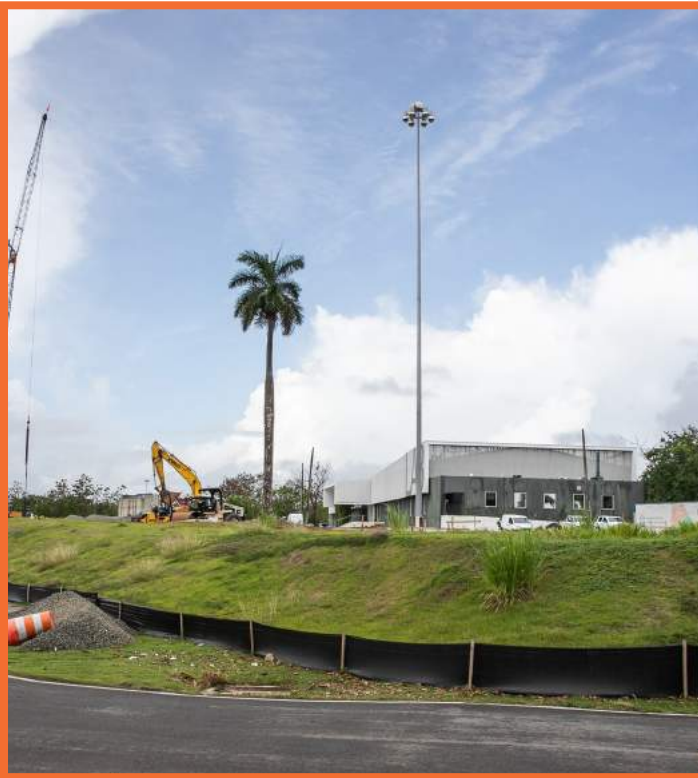
Forward Center Construction Process
